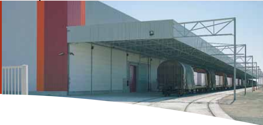
Entrepôt embranché fer A warehouse connected to the railroad network
